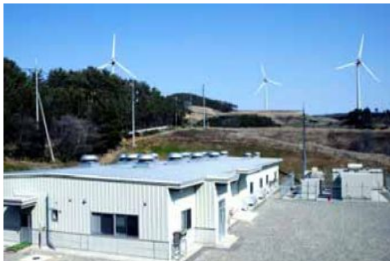
Wind turbine generator
