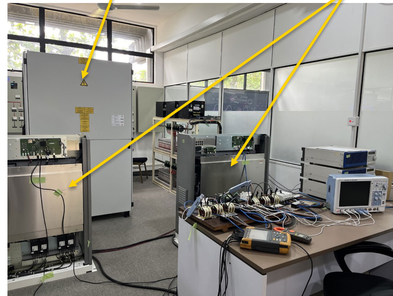
Newly Installed Digital Grid Research Lab
