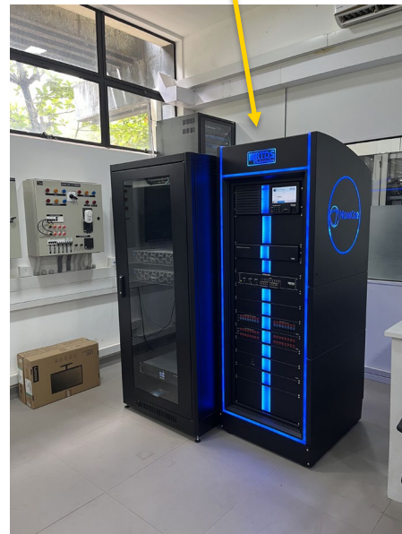
Existing LECO-UOM Smart Grid Research Lab
